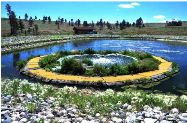
Figure 4 – Aerated lagoon with AFIs at Rehberg Ranch, USA (Floating Island International Inc. USA (2011))
