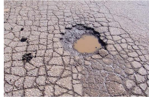
Figure 4.1 (b) Pothole
