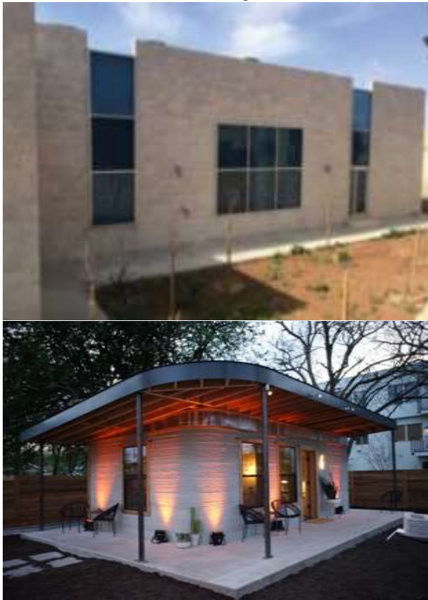
Fig.4. 3D Printed House [19,20] (Courtesy: The Verge)
