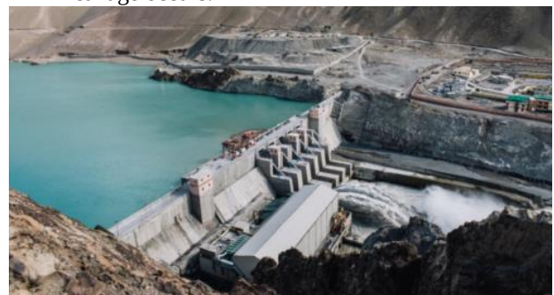
Fig.1. Dam Drainage observing.
