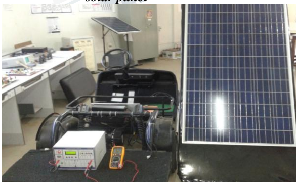
Figure.3: SiC Boost converter & 250 W Solar panel Battery charging setup
