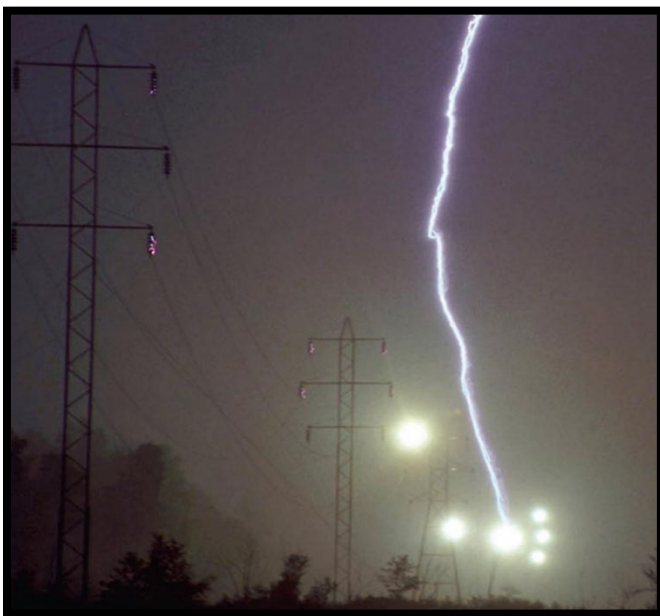
Fig2. Back flashover in transmission lines during lightning
