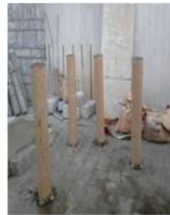
d) Casting of columns
