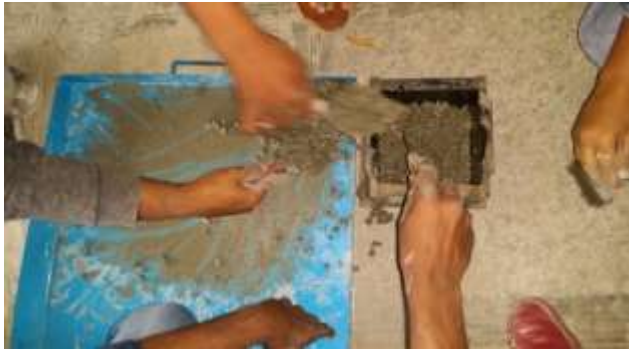
Moulding the pervious concrete after greasing the mould to easy removable of cube.
