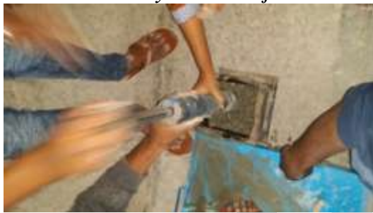
Compacting the concrete into
