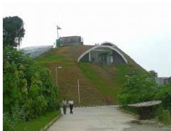
Fig 2. ONGC Green Roof
