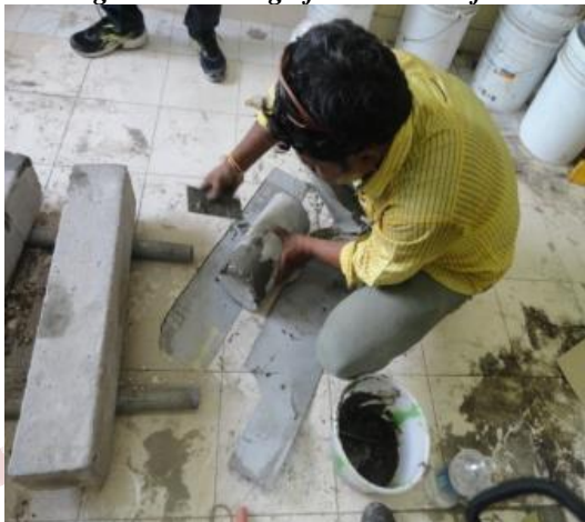
Figure 2 filling the holes with cement plaster
