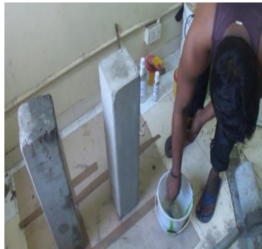
Figure 4 Mixing of chemicals
