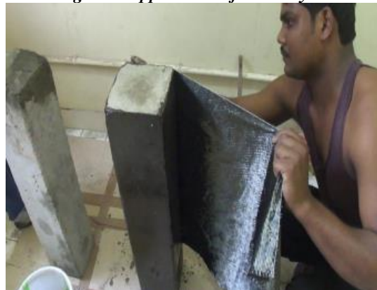
Figure 6 Application of carbon fiber material
