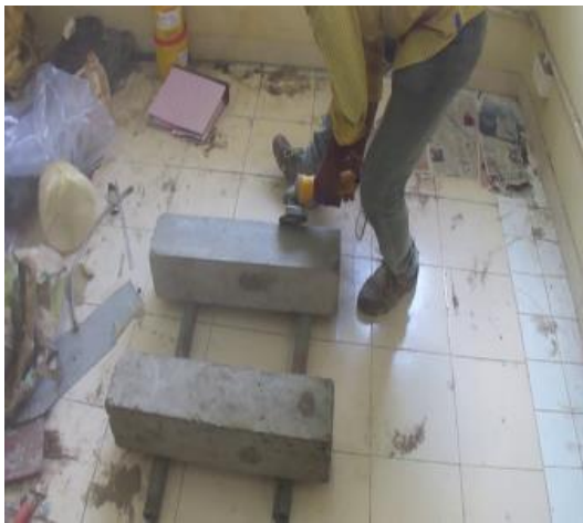
Figure 1 Grinding of concrete surface
