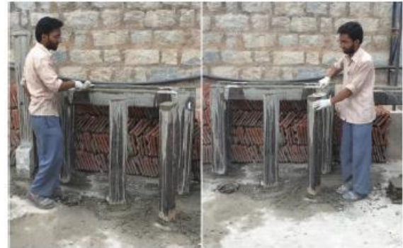
Fig 2: Finishing to the concrete exposed surfaces of frames and column.
