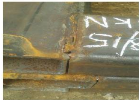
Fig 10: Connection failure of the specimen HSTF-01
