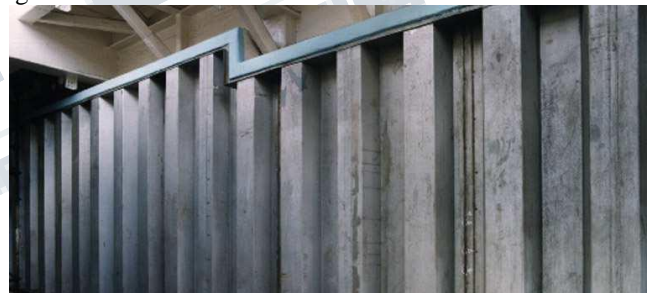
Fig. 5. Existing blast walls of an offshore platform [13]
