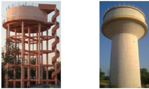
Fig. 1 Staging types (a) RC frame type of staging, (b) RC shaft type of staging
