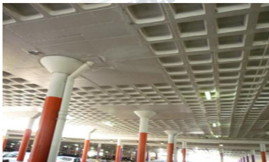
Figure 3d. Waffle Slab with Column head. (Source http://sketchucation.com )
