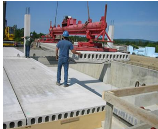
Figure 6b. Precast Hollow Core Slab (Source http://www.jpccarrara.com ) Figure 6. Precast Slab
