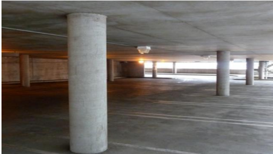
Figure 1a. Flat Plate Slab resting directly on Column (Source https://www.nexus.globalquakemodel.org )
