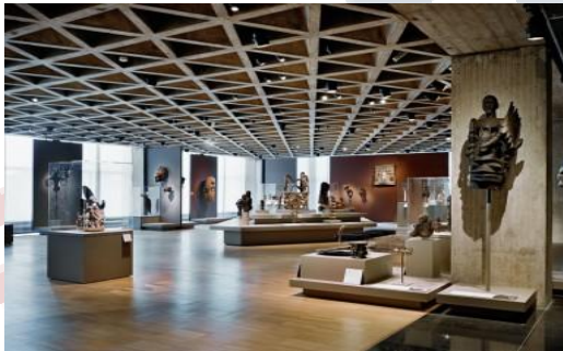
Figure 3c. Waffle / Ribbed Slabs (Source http://www.worldarchitecturenews.com )
