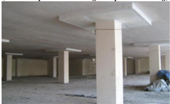
Figure 1b. Flat Slab with Drop Panels
