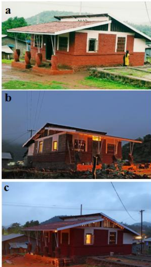
Fig.10 (a,b,c) Completed Dwelling unit at Dasgoan.
