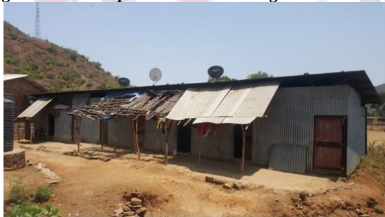
Fig.3: Temporary shelters Dasgoan
