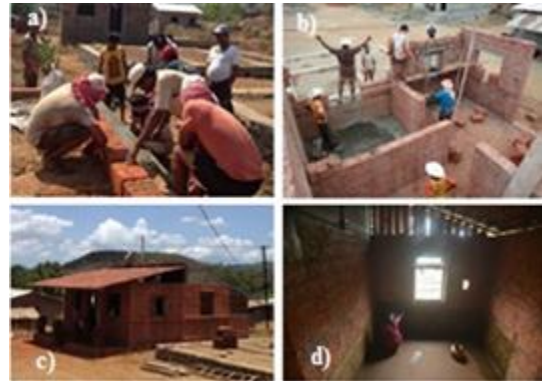
Fig.9: Image showing the construction process (a,b,c,d) showing Construction of plinth beam,
