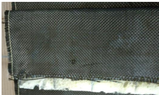
Fig 12: Blade after wrapping to Carbon Fiber
