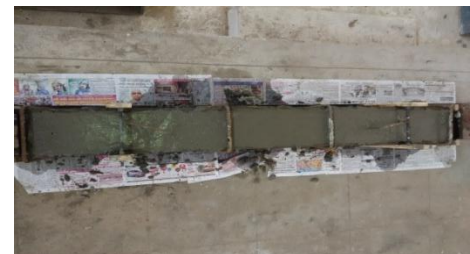
After Casting Of Beam
