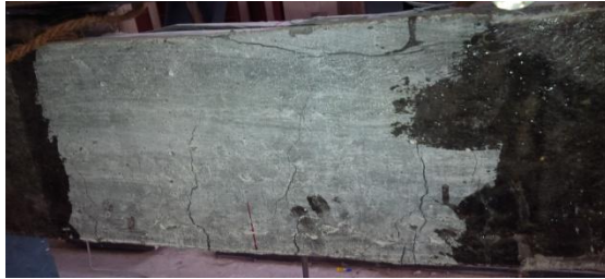
Ultimate failure of strengthened beam 2
