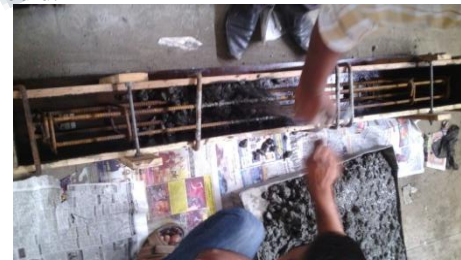
During casting of beam
