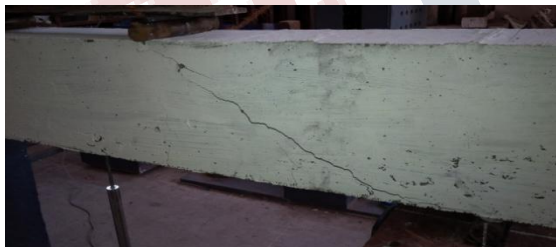
Ultimate failure of control beam
