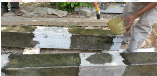
strengthening of beams with GFRP sheets
