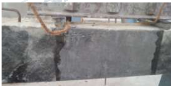
Ultimate failure of strengthened beam 3
