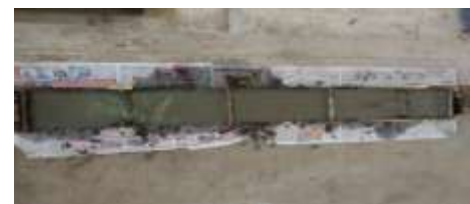
After Casting Of Beam
