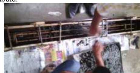
During casting of beam
