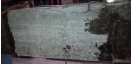
Ultimate failure of strengthened beam 2
