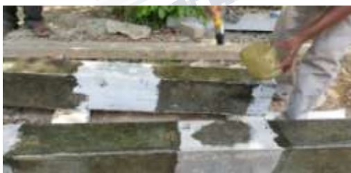
strengthening of beams with GFRP sheets
