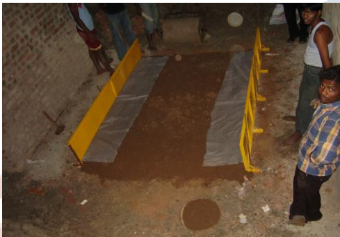
Plate 1. Wrapping with geotextile layer over the compacted fill within the lift thickness
