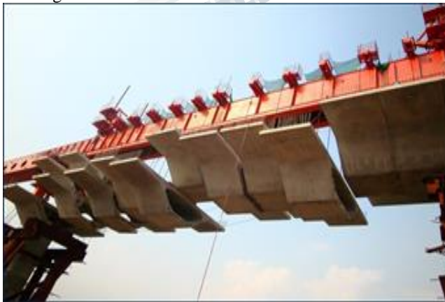
Fig.1 Post-tensioned precast segmental bridge (source- http://sunengineering.cn )
