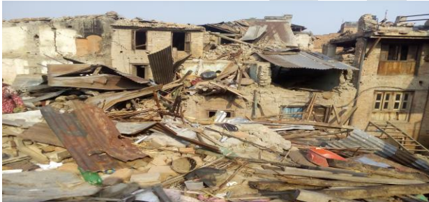
Fig. 7. Damages seen at Jellan, Bhaktapur.
