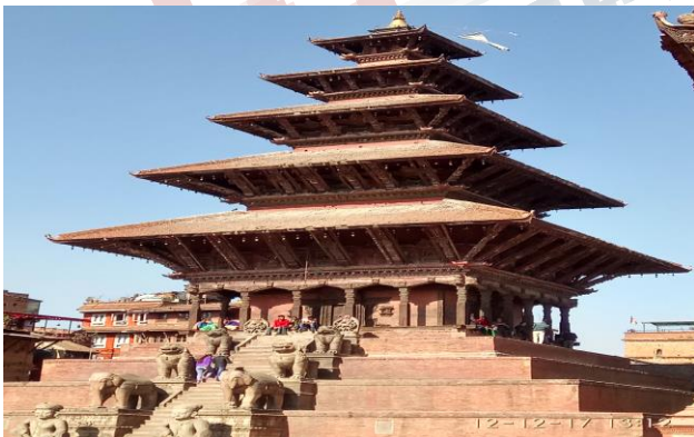
Fig. 8. Minor Damages in the World Heritage, Naytapolan.
