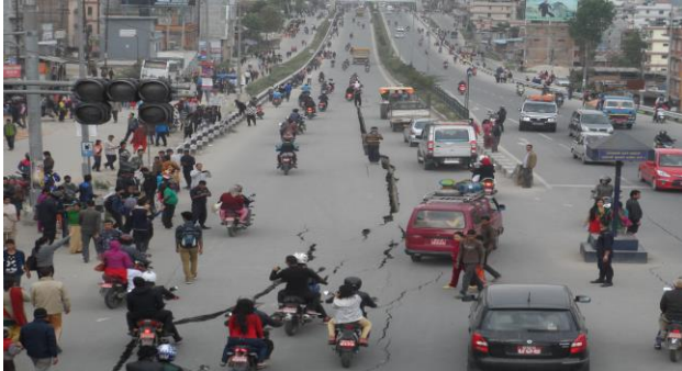
Fig. 3. Damaged road at Kausaltar, Bhaktapur
