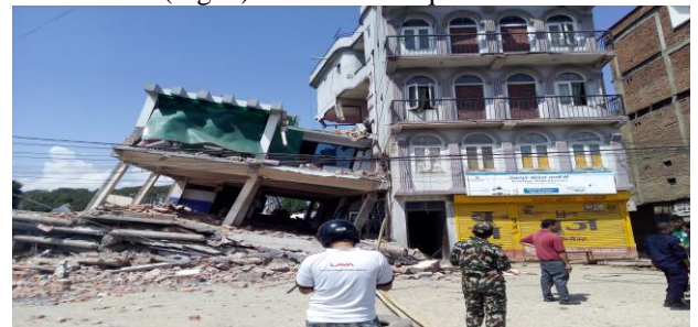
Fig. 2. Collapsed RC Frame Buildings at Bhaktapur -17 due to aftershock on 12th May 2015
