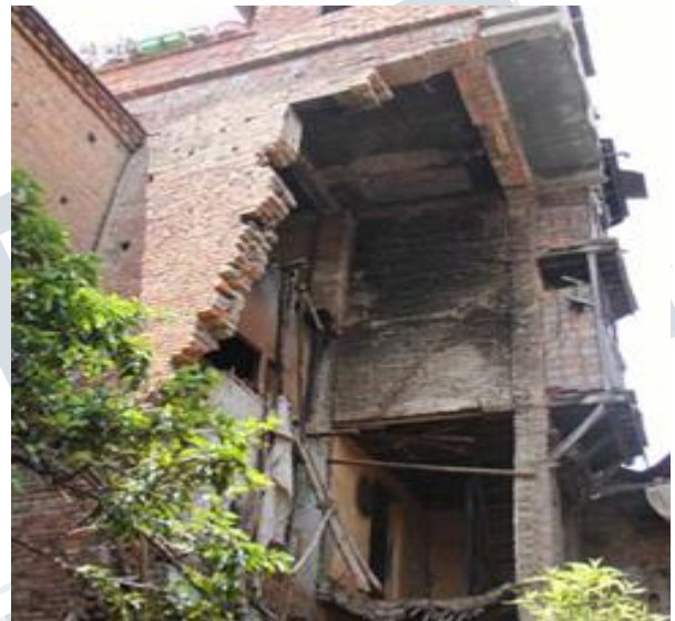
Fig. 9. Hanging Non Engineered Modification house (Source: BM).
