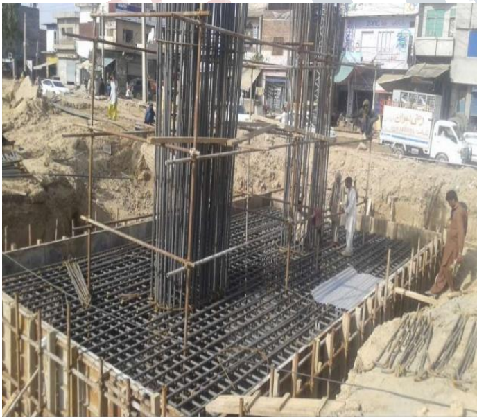
Figure 2 : Pile foundation for flyover
