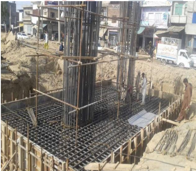
Figure 2 : Pile foundation for flyover
