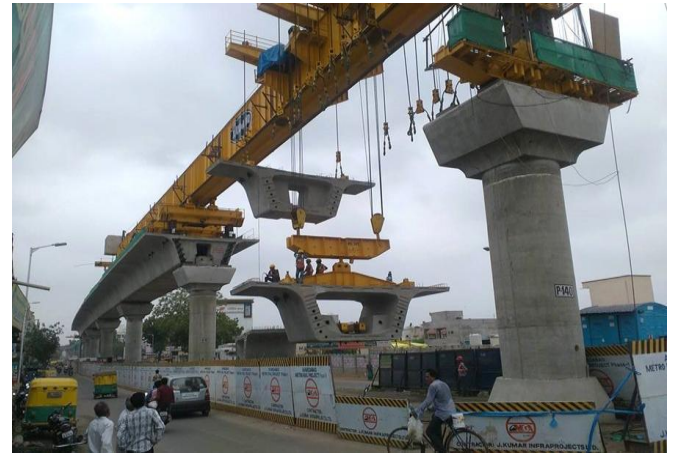
Figure 3 : Circular piers used in flyover construction
