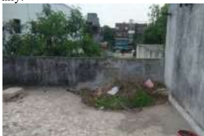
Fig. 6 “Growing shrubs and debris”
