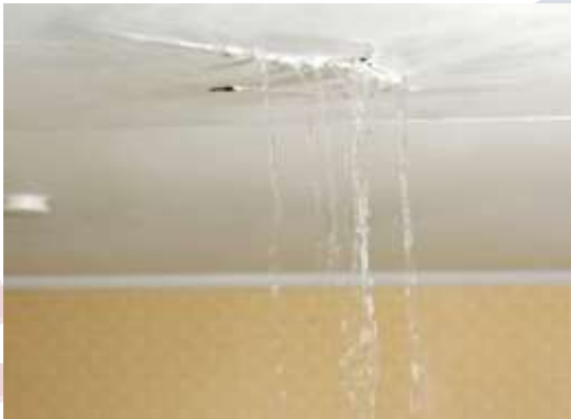
Fig. 5 “Slab leakage”
