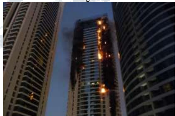
Fig. 4 “Neglected Building Services”
