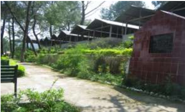
Figure 3 Solid Waste Management Plant Hamirpur, Himachal Pradesh, India
