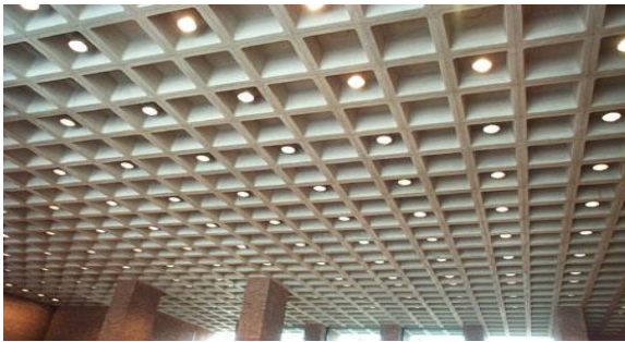
Fig 1.3 Waffle slab
