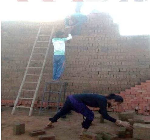
**Fig. 8. Transferring the Sun dried brick into kiln burning**
