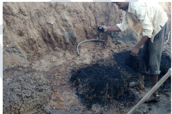
**Fig. 4. Covering of kneaded mud with fly ash**
