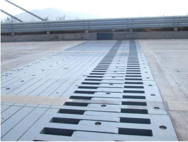
Figure 10: Expansion Joints
