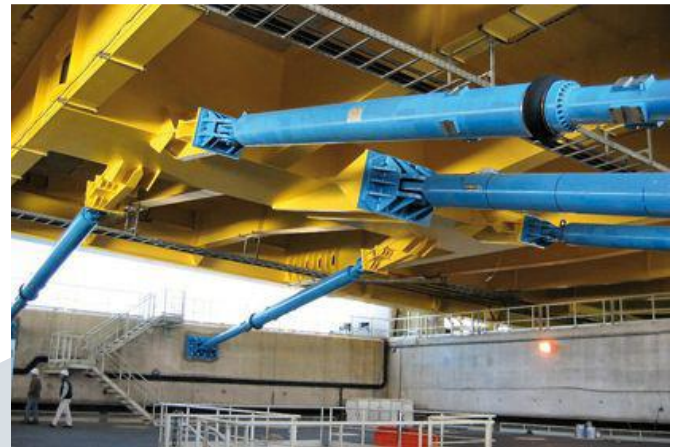
Figure 6: Viscous Dampers
