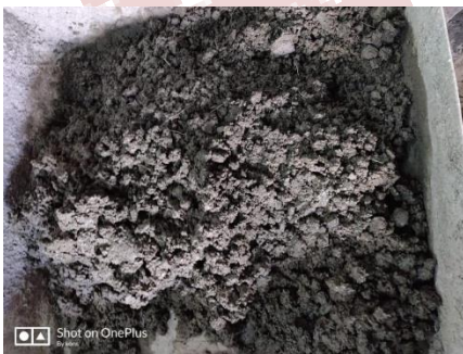
Mixing of concrete
