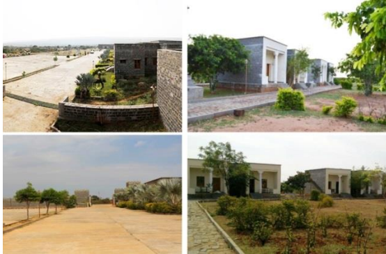
Fig. 9. Gandikota APTDC complex-heritage resort
