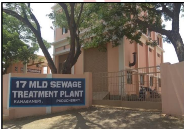
Fig. 1- Kanaganeri Sewage Treatment Plant
