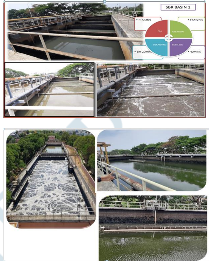
Fig.2- Kanaganeri Sewage Treatment Plant interior elevation
