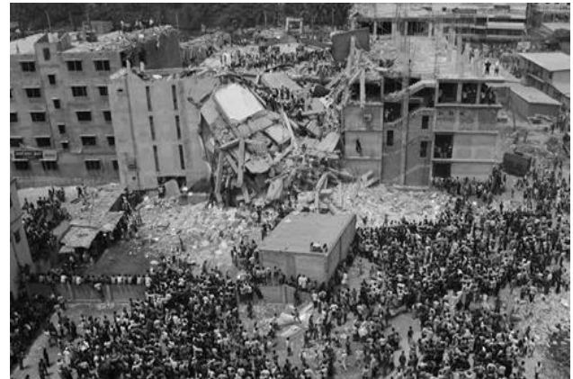
Fig 7: Bangladesh Building Collapse [11]
