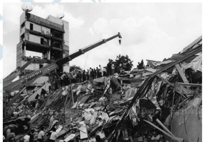
Fig 4: Royal Plaza Hotel collapse [7]
