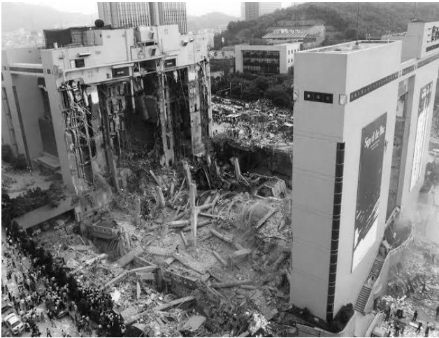
Fig 5: Sampoong Department Store collapse [9]
