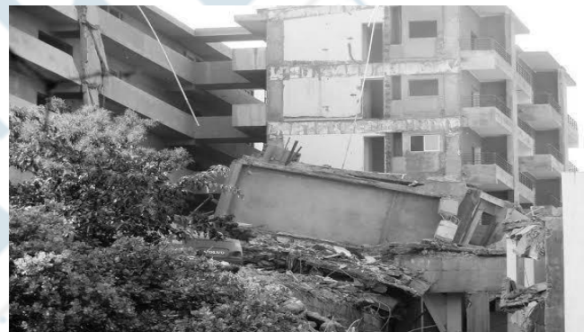
Fig 8: Residential building collapse [12]
