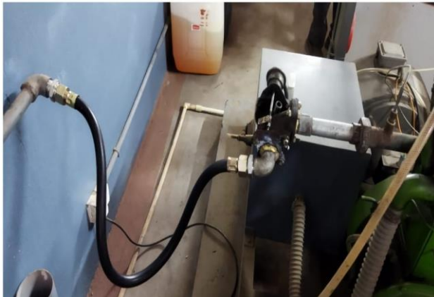
FIG 1. Experimental setup of waste heat recovery
