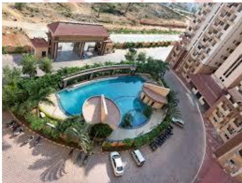
Fig. 5 Swimming pool View from top floor
