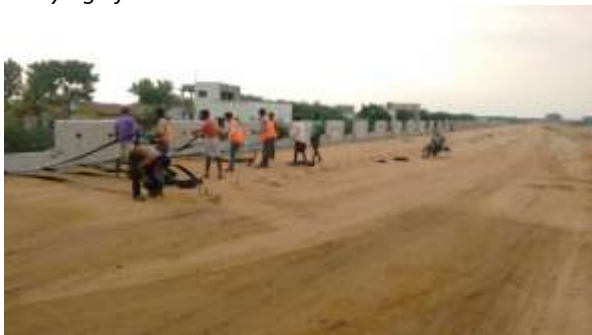
Laying of ParaWeb
