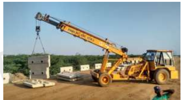
Erection of Panels
