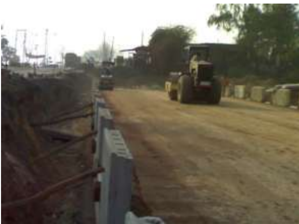
Rolling and compaction of soil
