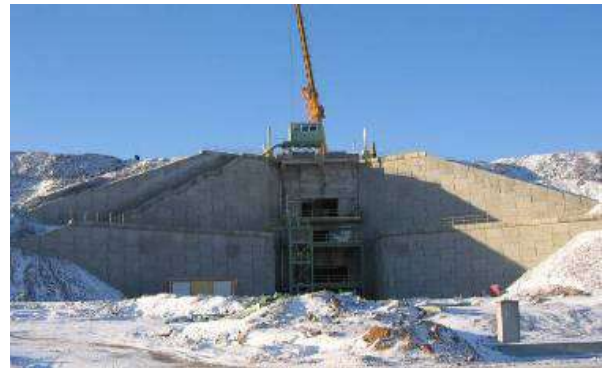
Crusher Plant (Crusher walls)
