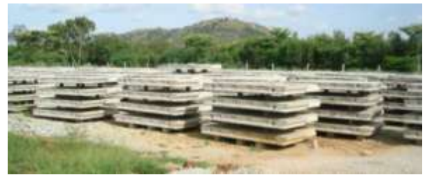
Stacking of Panels
