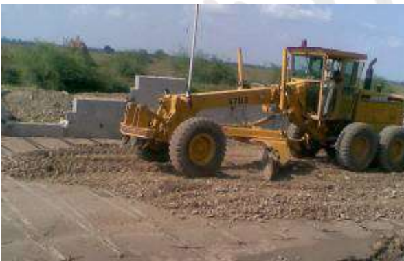
Grading of Fill Material
