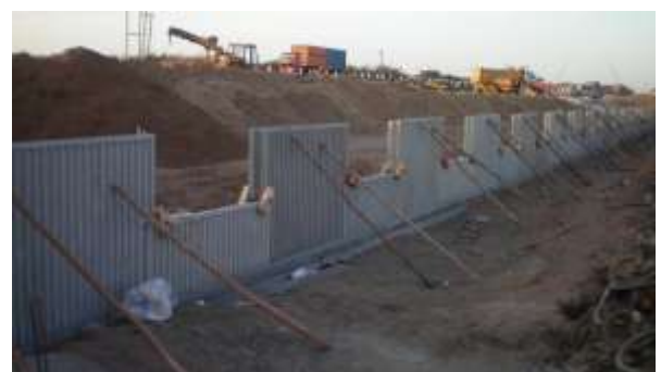
Timber supports to prevent over-turning
