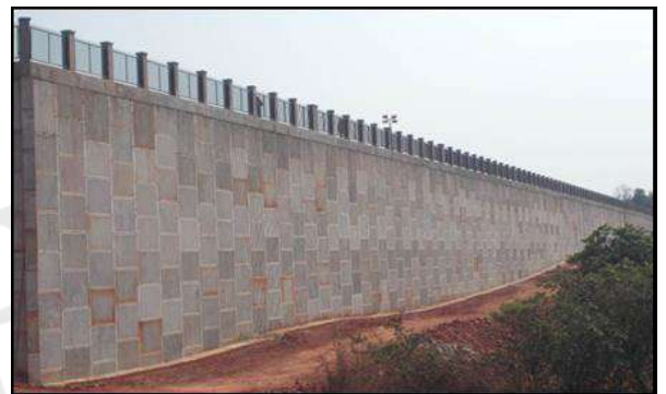
Building Sector (Boundary walls)
